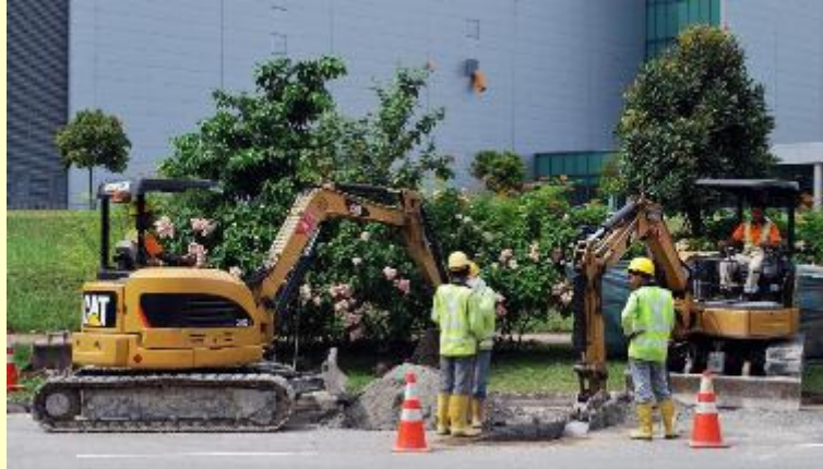
A pair of Cat 304 preparing the road for the pipes to be laid.
