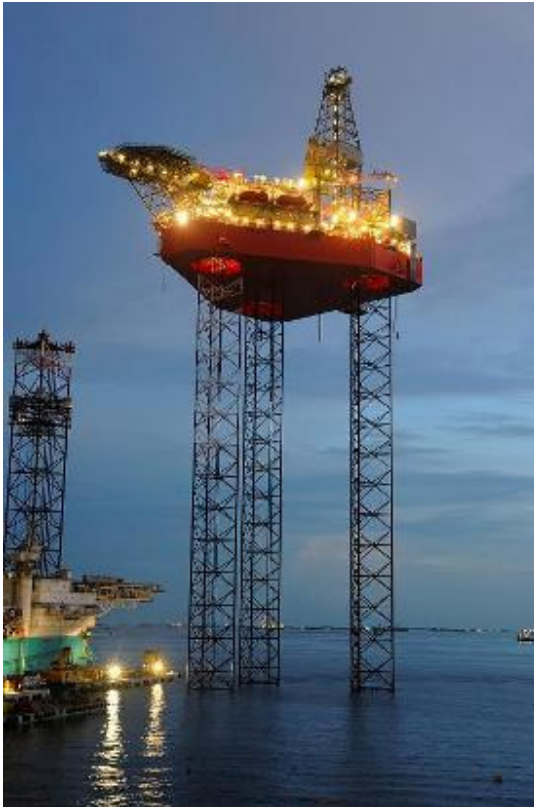
West Callisto – the 32nd KFELS B Class jackup rig to enter the market
