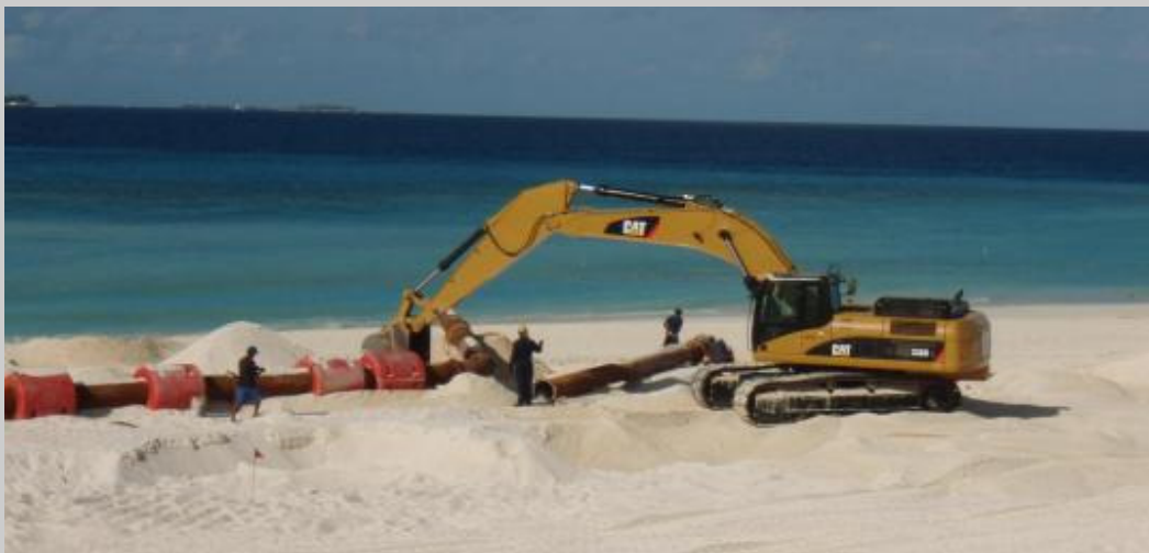
Land reclamation works at K Bolifushi Resort Development Project
