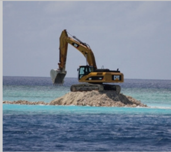
Harbour reconstruction works at Raa Meedhu Island
