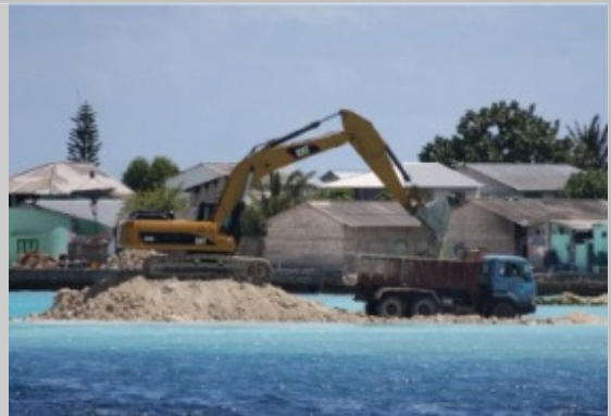
Harbour dredging works at Raa Meedhu Island
