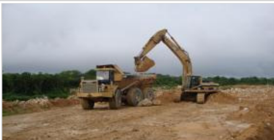
Cat Hydraulic Excavator 330BL loading phosphate into a Cat D400E dumptruck.
